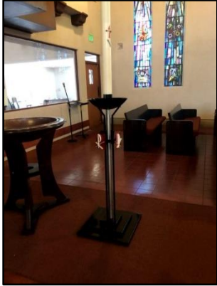
Skip installed the new half pews, made from the originals, but shortened to leave room around the new font.
